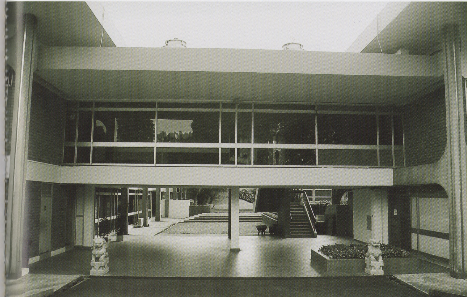
Link bridge used to house the secretaries' offices between the interlocking blocks, allowing visually and physical continuity between the courtyard and its surroundings.
