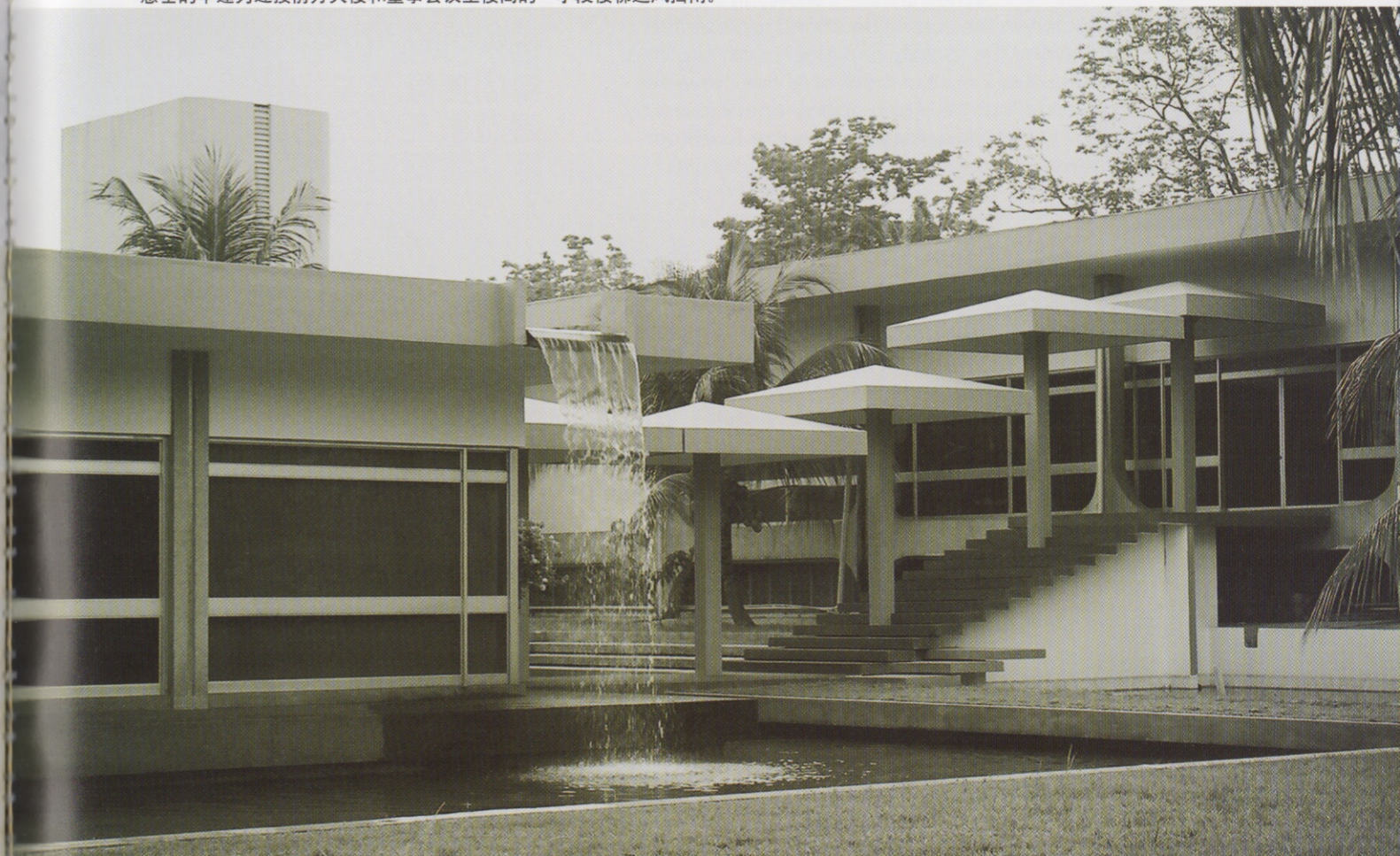
Cascading umbrella canopies shelter a short flight of stairs which connects the front block to the boardroom pavilion. 悬垂的伞篷为连接前方大楼和董事会议室楼阁的一小段楼梯遮风挡雨。
