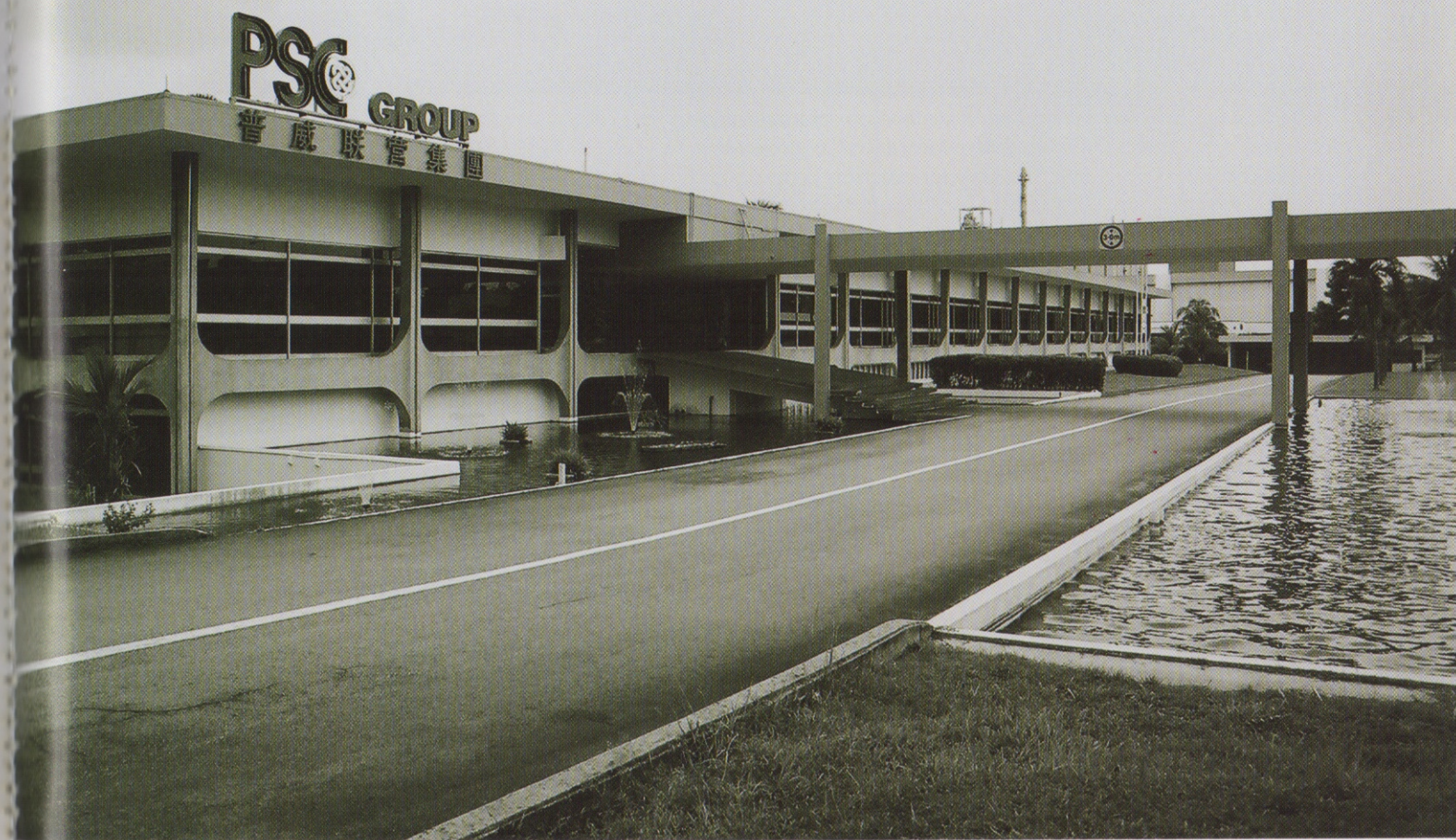
Public face of the FEP building, with an extended porch over the driveway. Visitors enter the complex via a raised sloped bridge over a reflecting pool. 远东印刷厂建筑正面的门廊横跨于车行道之上。来访者登上横跨倒映水池的坡道桥进入该建筑群。
